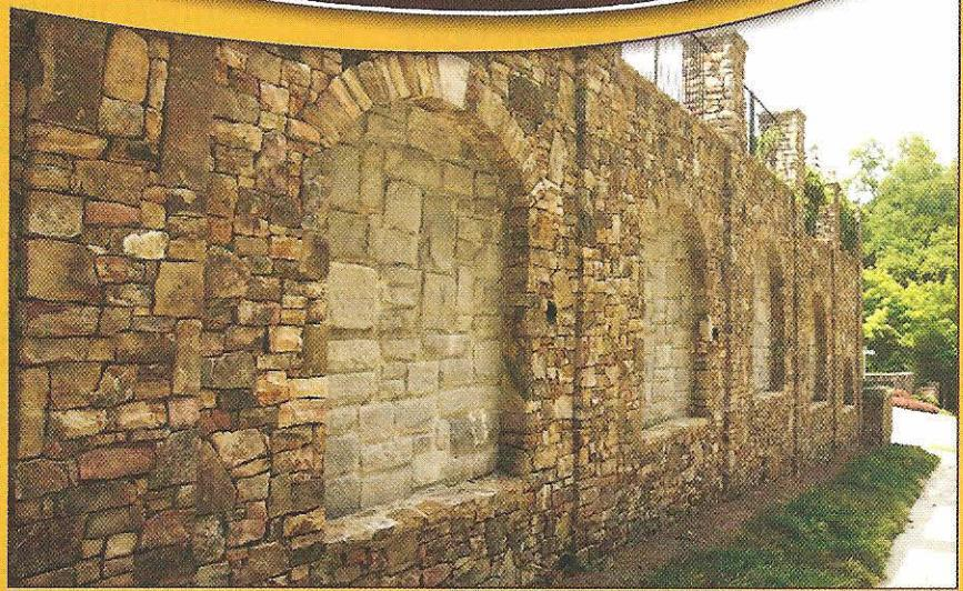
This new product is easy to install and allows you to attach Natural Stone to the geo grid technology of today. The geo grid has the same connection strength from the top to the bottom of the wall. Once the mortar mix dries, the geo grid becomes Mechanically Connected to the natural stone facing. The wall is *Static* which creates virtually no cracking or movement. Build your walls with strength and beauty.
